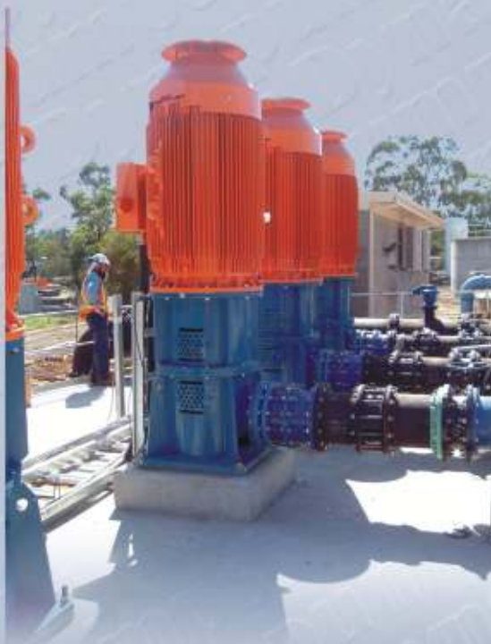
Flo-Max Turbine pumps installed for Town Water Supply Dubbo, NSW
