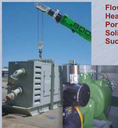
Mine de-watering pump in acoustic enclosure
