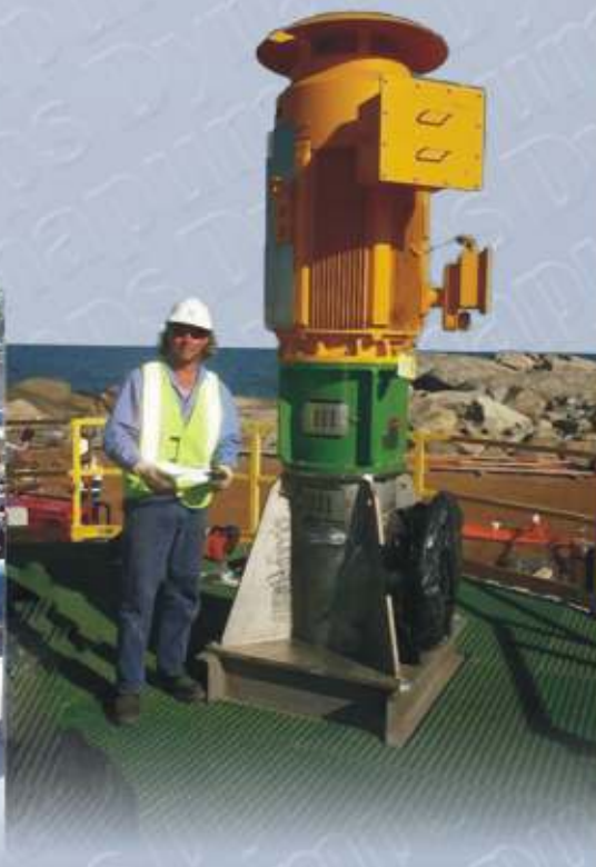
One of nine Super Duplex Flo-Max Turbine pumps pumping seawater at Nickel Mine in Ravensthorpe, W.A.
