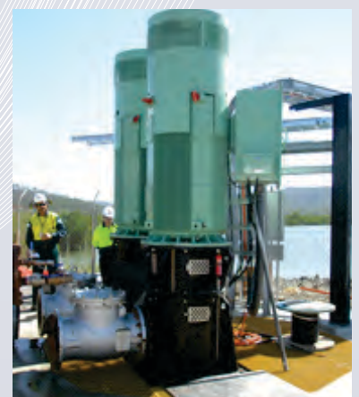
Water supply from dam
