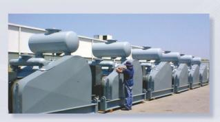
315 kW, 4,000 Nm³/h Pumps for Alumina Seed Filters – West Australia
