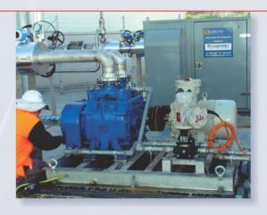
Compressor in Biogas (Methane) Digester Plant
