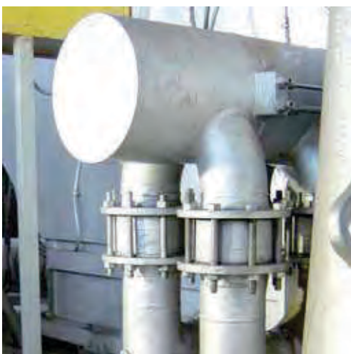
3 Reduction Gear Lube Oil Pump L3MG
