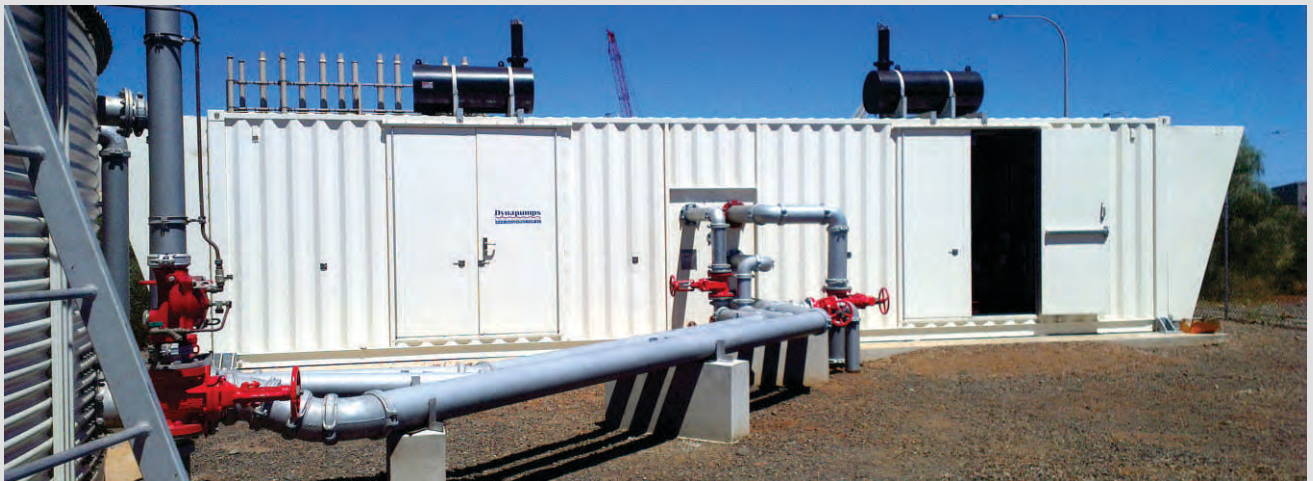
Above: Containerised Fire Pump on site Below: 3D rendering of the system
