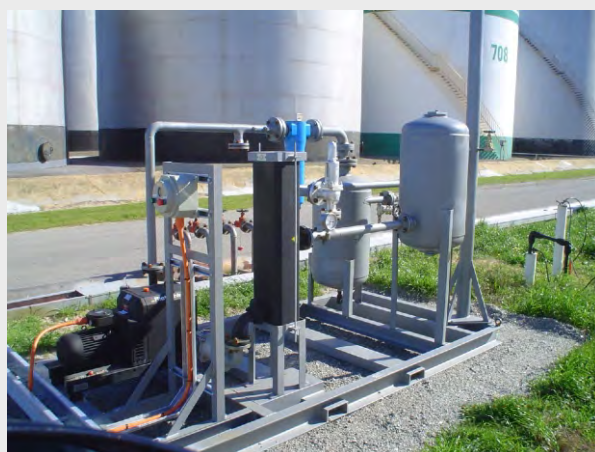
Claw Type Vacuum Pump Skid on site in Kwinana, WA
